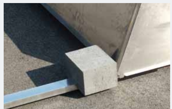
Ballasting at the periphery
